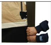
**4.** Grasp both sides of the bottom corners of the Corner Panel and pull slowly to remove the Corner Panel. The Corner Panel will be stuck to the foam insulation behind the Corner Panel and will require some force to separate from the foam. Some of the insulation foam will remain stuck to the Corner Panel.
